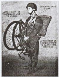
This one folds in half for a very special reason. It had to be made small so that men could carry it while jumping out of an aeroplane with a parachute. These men were called paratroopers. They had a parachute on their backs and a bicycle on their fronts. So when they landed on the ground they could jump on their bicycles and get to where they needed to be.
